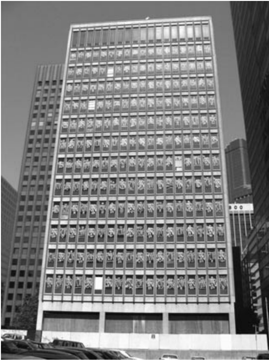
Figure 2 Office building, CBD, Melbourne. The windows on three sides of this building (those sides within public view) have been tagged in precise script. Each tag was written backwards (by two writers who were necessarily inside the building while putting up) so that work would be legible when viewed from the street. © Benjamin Pederick. Reproduced with permission.
